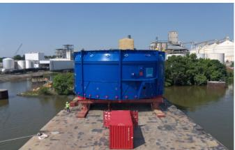
Upon arrival at site, the trucks were discharged straight to the holding area and the barge carrying the main unit was prepared for the rolling operation by placing the ramps to shore. After all was prepared, barge was balasted correctly, the unit was rolled off by way of two units SPMT.
