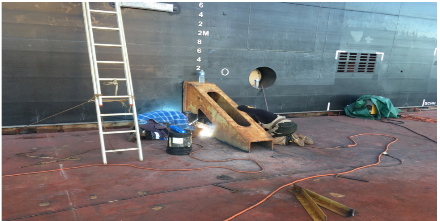
Specialist welding commences to secure the floating dock according to the seafastening plan
